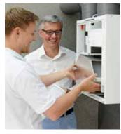
To maintain an optimised efficiency of the ventilation unit during its life cycle, Airflow recommends a filter replacement at least twice a year.
